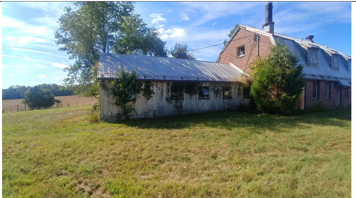
Exterior Elevation – North East End
