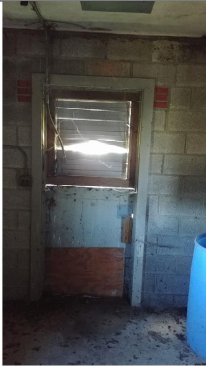
Interior – East End Addition
