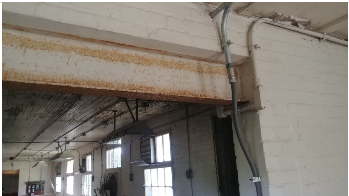
Original Interior Wall Was Removed
