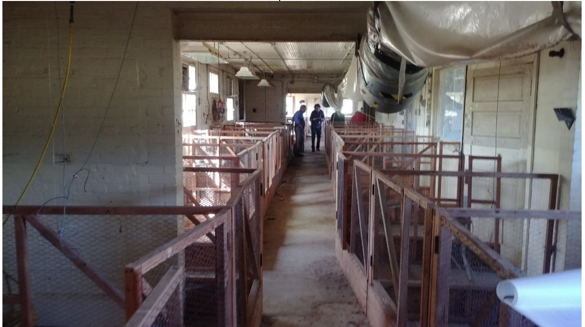
Interior – Looking West
