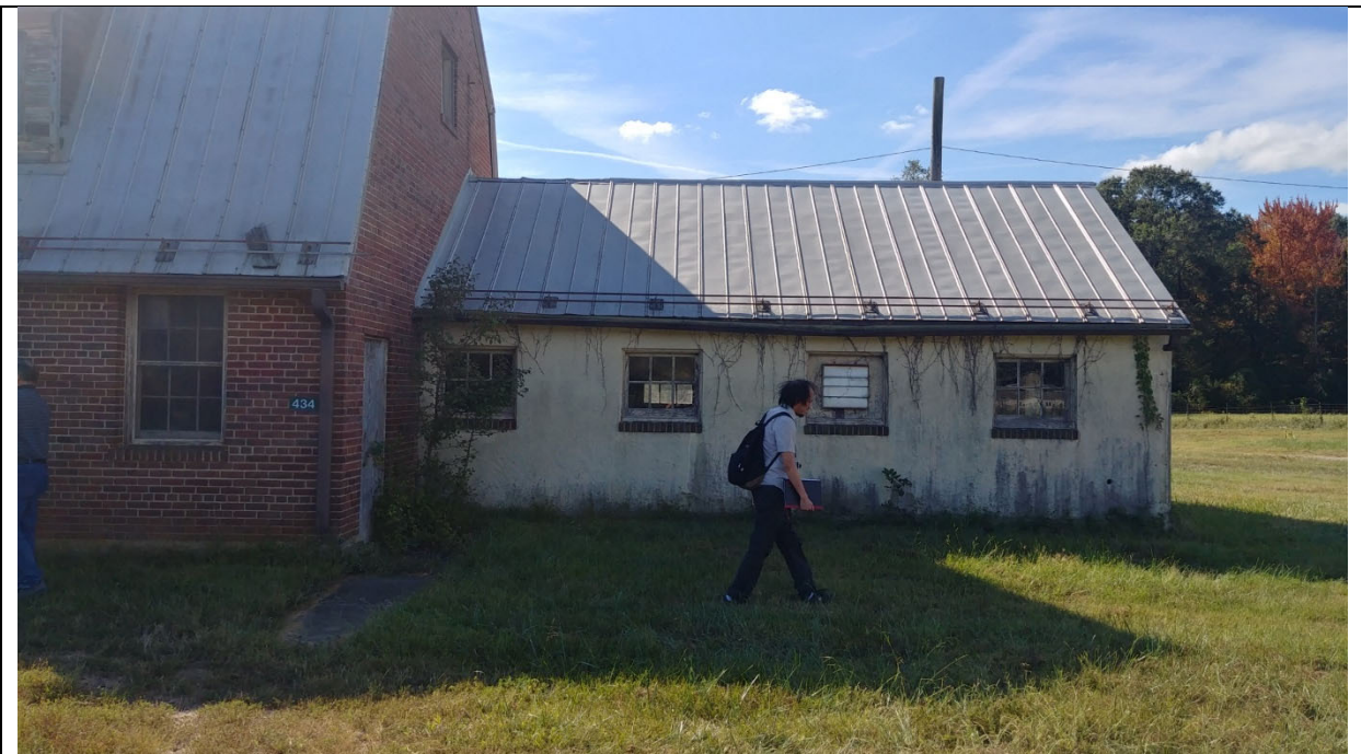
Exterior Elevation – North West End
